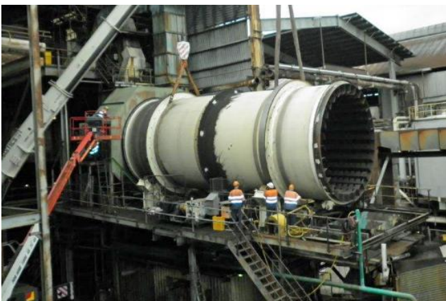
Installation of the drying drum for sugar
